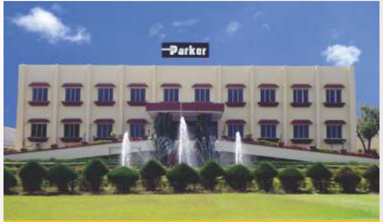
Hose Plant, Nagpur
